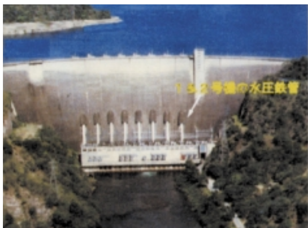
The Hydraulic Pressure Pipes, units 1 and 2
