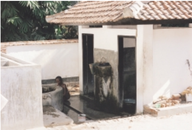
A Public Water System with a well, Toilets, a Bath and a Washhouse in a Remote Rural Village, Sumatera Utara
