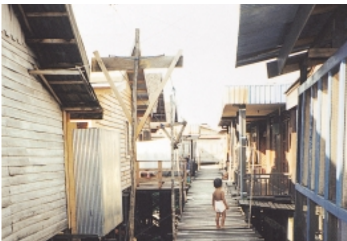
Provided Access Roads in Kalimantan Timur
