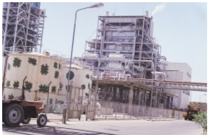
A View of the Jamshoro Thermal Power Station showing Boiler and Turbine Building in the Background
