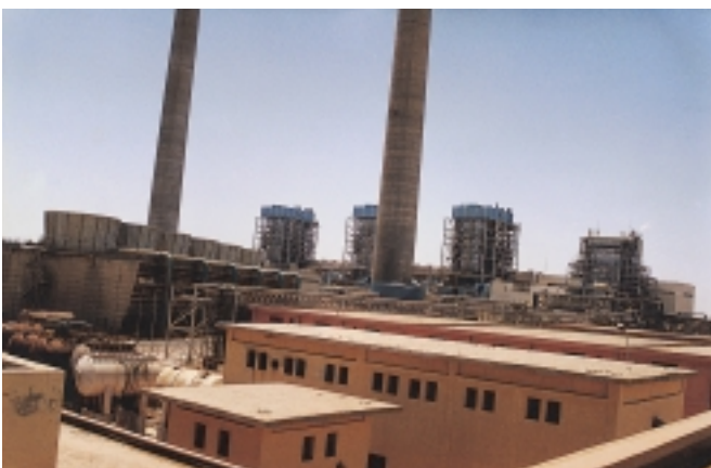
A View of the Jamshoro Thermal Power Station, Cooling Tower on the Left.
