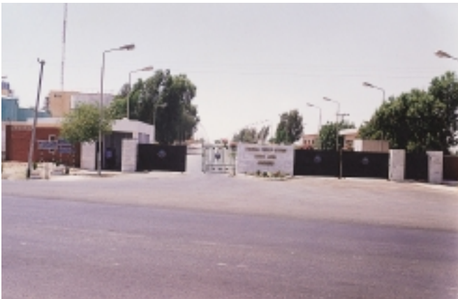
Main Entrance of the Jamshoro Thermal Power Station
