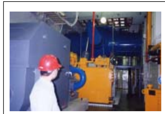
Shisanling Pumped Storage Power Station
