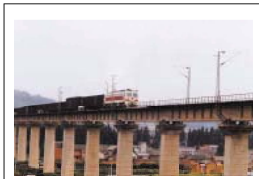
Bridge between Kunming and Kunming South, Nankun Line
