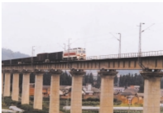
Bridge between Kunming and Kunming South, Nanning-Kunming Line
