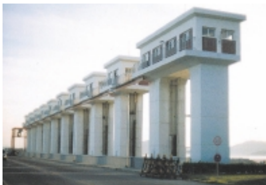
Tidal Barrage constructed by the Project
