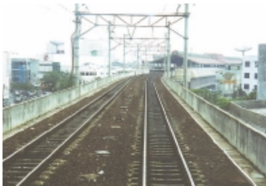
Section of Track Elevated by the Project
