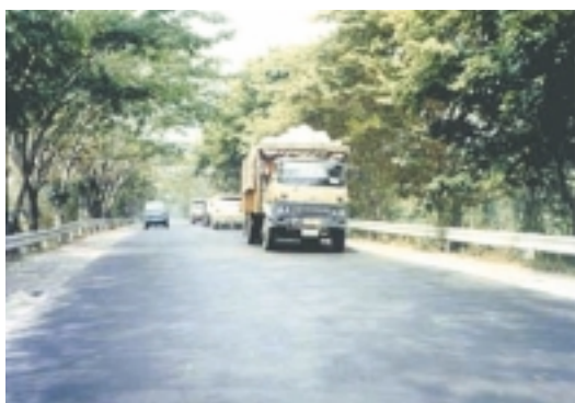
Rehabilitated Section in Lampung Province, Sumatra
