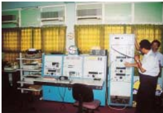
SAR Telecommunication Equipment
