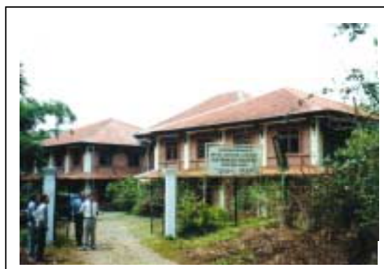
Maintenance Center in the Suburb of Jakarta
