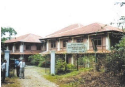
Maintenance Center in the Suburb of Jakarta
