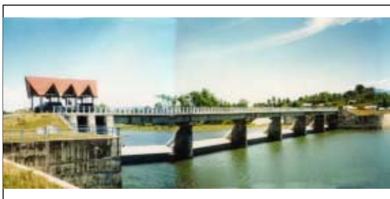
Headwork Constructed by this Project
