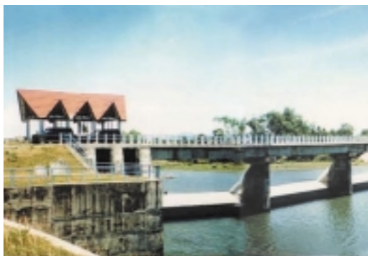
Headwork Constructed by the Project
