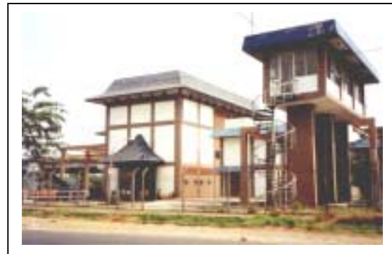
Ancol Drainage Facilities
