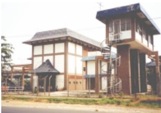
Ancol Drainage Facility
