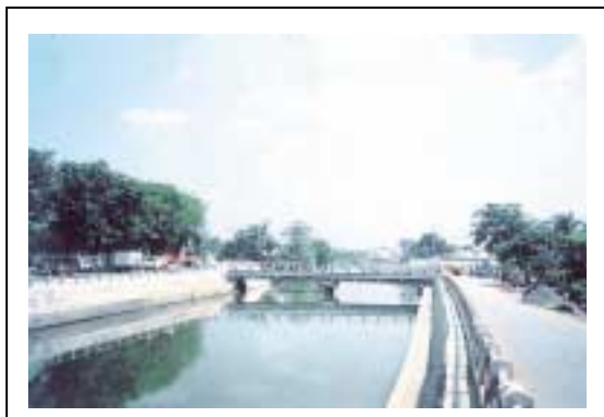
River Wall Rehabilitated by the Project (near Jogoroyo Bridge)
