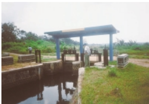
Primary Channel Gate
