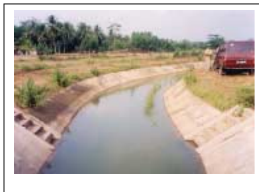
Trunk Canal of the Project Area
