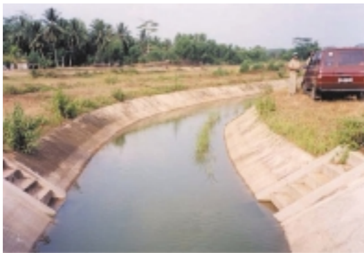
Trunk Canal of the Project Area
