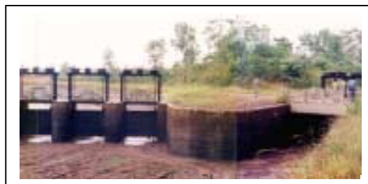
Water Distribution Junction (right) from Trunk Canal (left)
