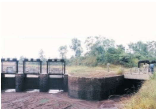
Diverging Point of Water Distribution (right side) from Trunk Channel (left side)
