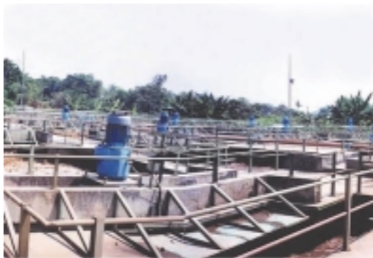
Overall View of Water Treatment Facilities
