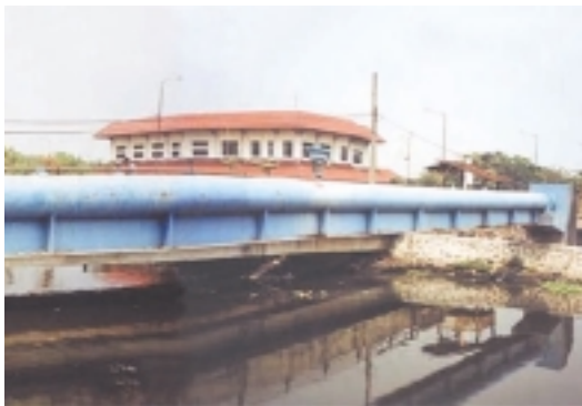
Distribution Pipeline Laid by the Project
