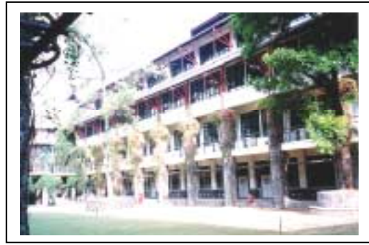
School Building Newly Constructed by this Project (No.5 Building)
