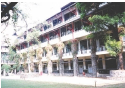
School Building newly Constructed by the Project (No.5 Building)
