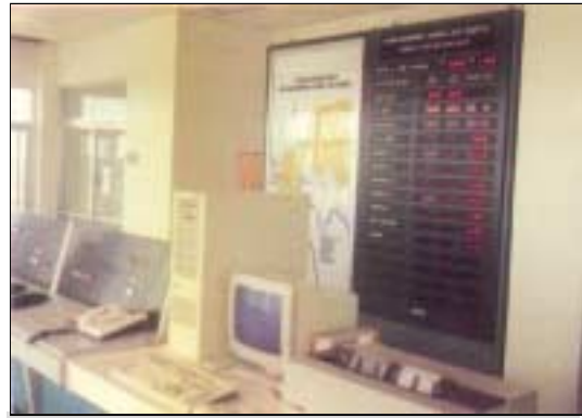
Rosario Central Monitoring Facility
