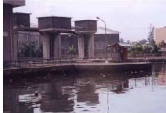
Bitas Pumping Station
