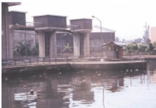
Vitas Pumping Station
