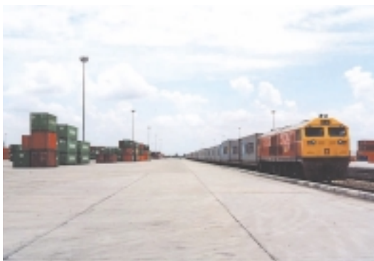
Inland Container Terminal, Lat Krabang Station
