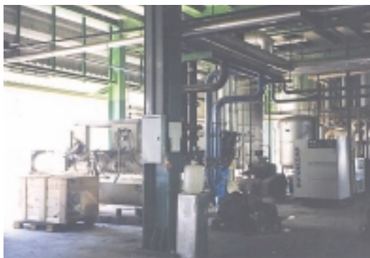
Valve Factory (Panton Thani Area)
