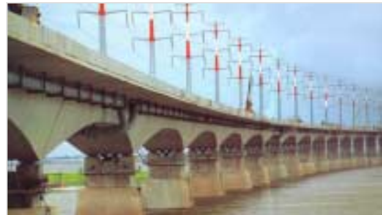
Jamuna Multipurpose Bridge
