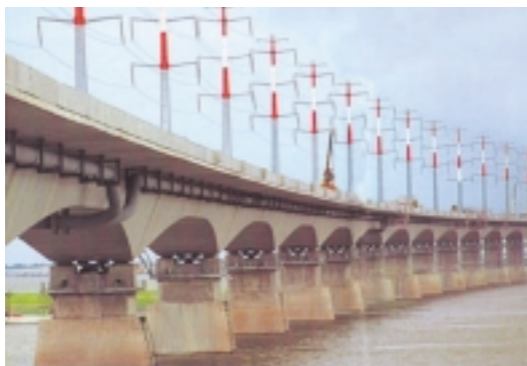
Jamuna Multipurpose Bridge
