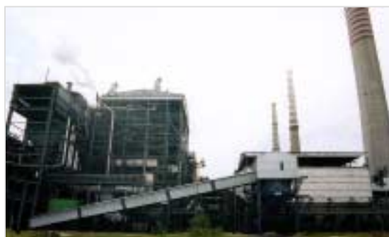
Raichur Thermal Power Plant
