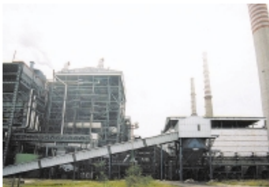
Raichur Thermal Power Station
