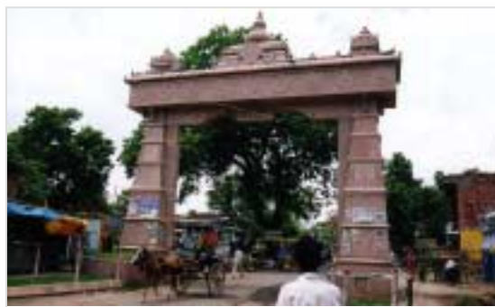
Photo: The entrance gate at Nalanda
