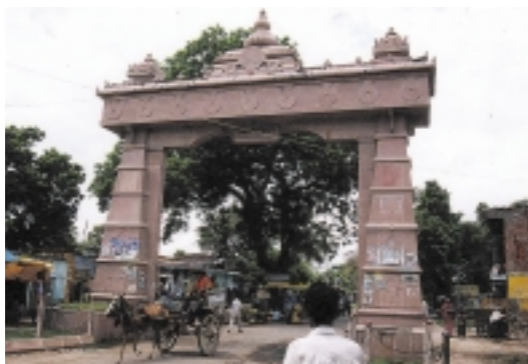
Entrance Gate Constructed in Nalanda
