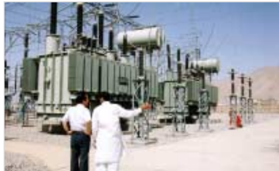
Photo: Industrial II Substation
