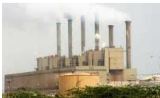
Site Photo: Bin Qasim Thermal Power Station
