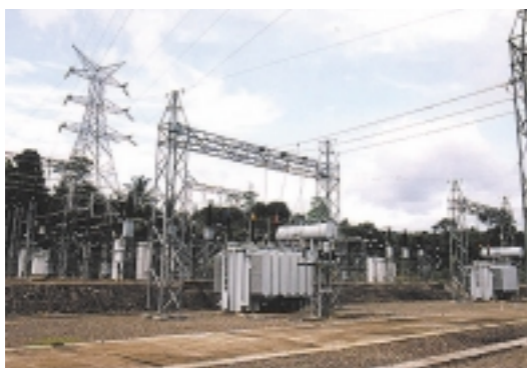
Avissawella Transformer Station
