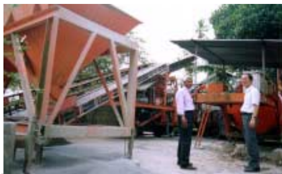
Equipment procured under the project
