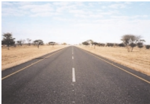
Trans-Kgalagadi Road Constructed by the Project
