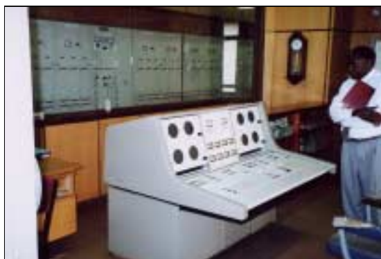
The KBC Ngong Transmission Station in suburban Nairobi
