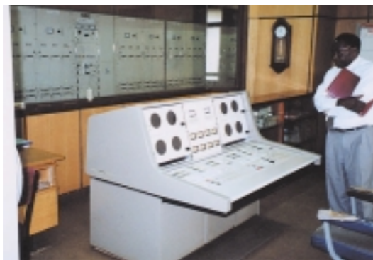
KBC Ngong Transmissiion Station (at the suburb of Nairobi)
