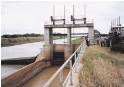
Tana Delta Irrigation, Sailoni Headwork
