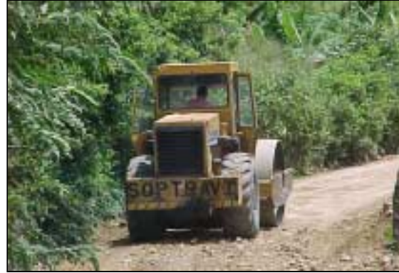
Procured equipment in use
