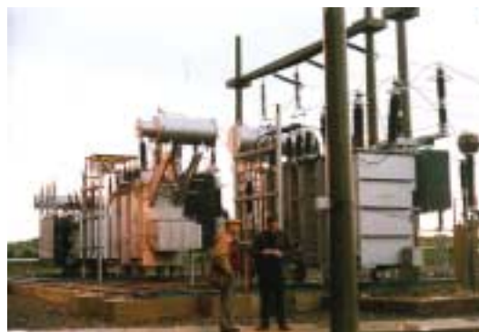
Facilities installed under the Project
