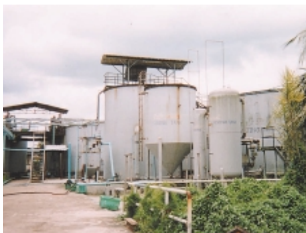
Waste Water Treatment Equipment in a Food Processing Factory
