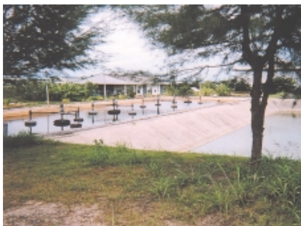
Waste Water Treatment Equipment in an Industrial Park
