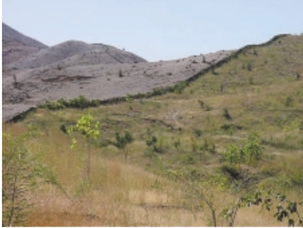
Forest land (foreground) Revived by the Construction of a Protective Wall
