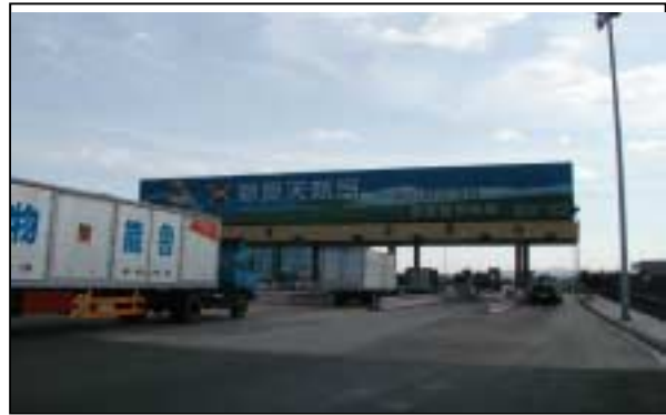
Site Photo: Guanjialou Tollgate of Jiaozhou Bay Expressway
